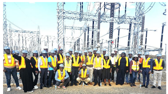
SAPP TWG Members at Phombeya substation
