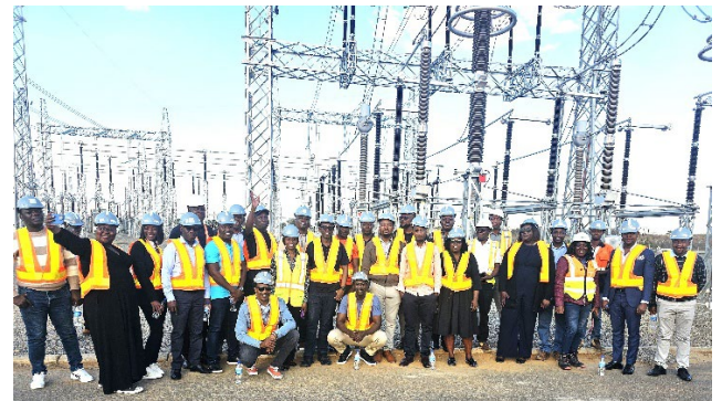
Some TWG Members at Phombeya Substation in Malawi
